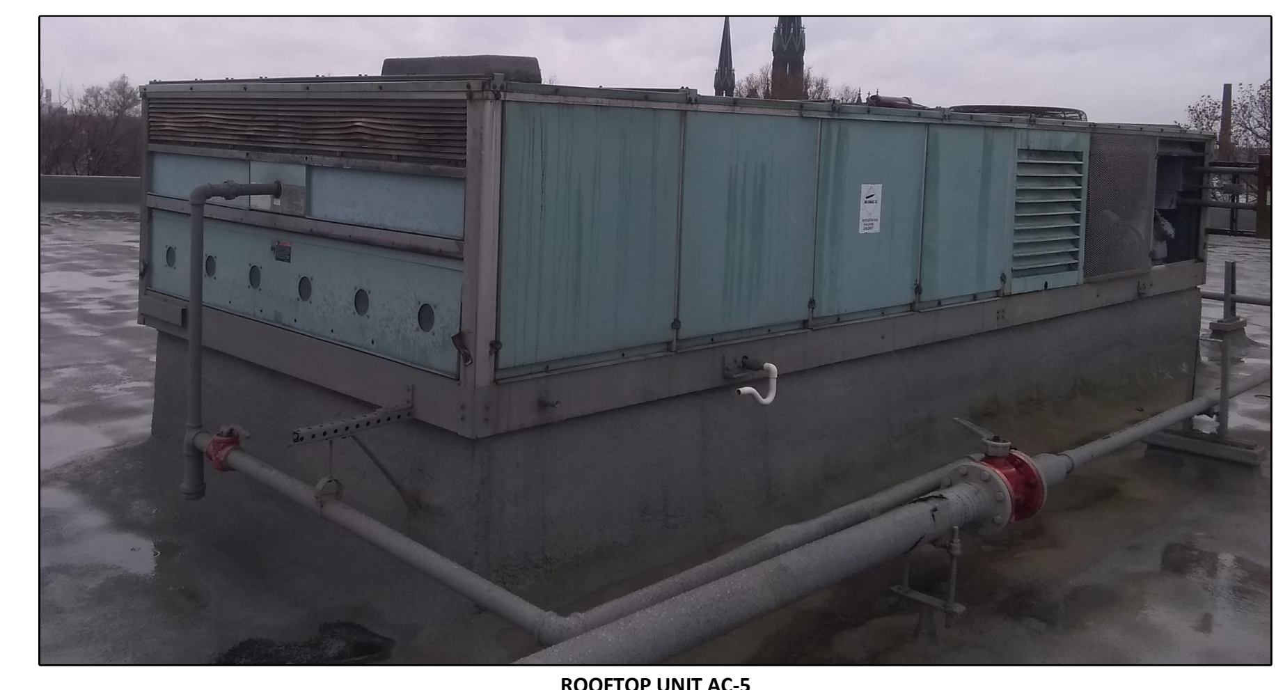
ROOFTOP UNIT AC-5
